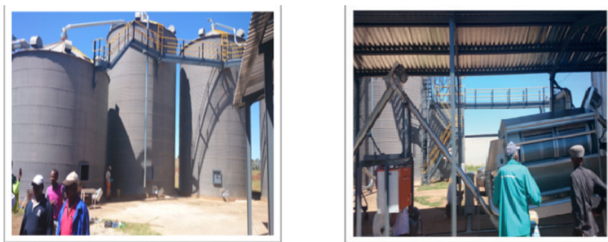
FIG.12 Silos at Qamata Agricultural Cooperative in Cofimvaba (Eastern Cape) funded through CASP
